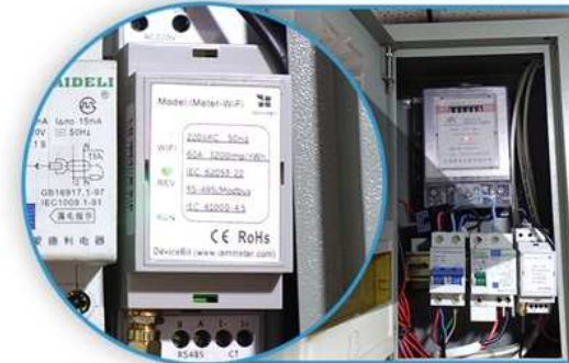
After iMeter Installed
